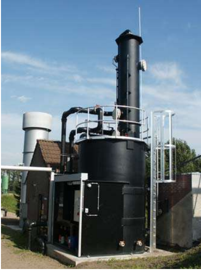
Figure 8.3 Hydrogen Sulfide Scrubber (courtesy of Tetra Tech)
